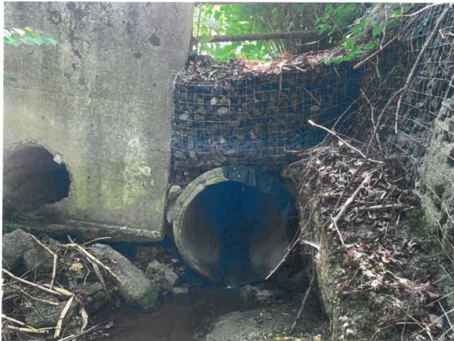
Figure 4 – Concrete Outlet Pipe
