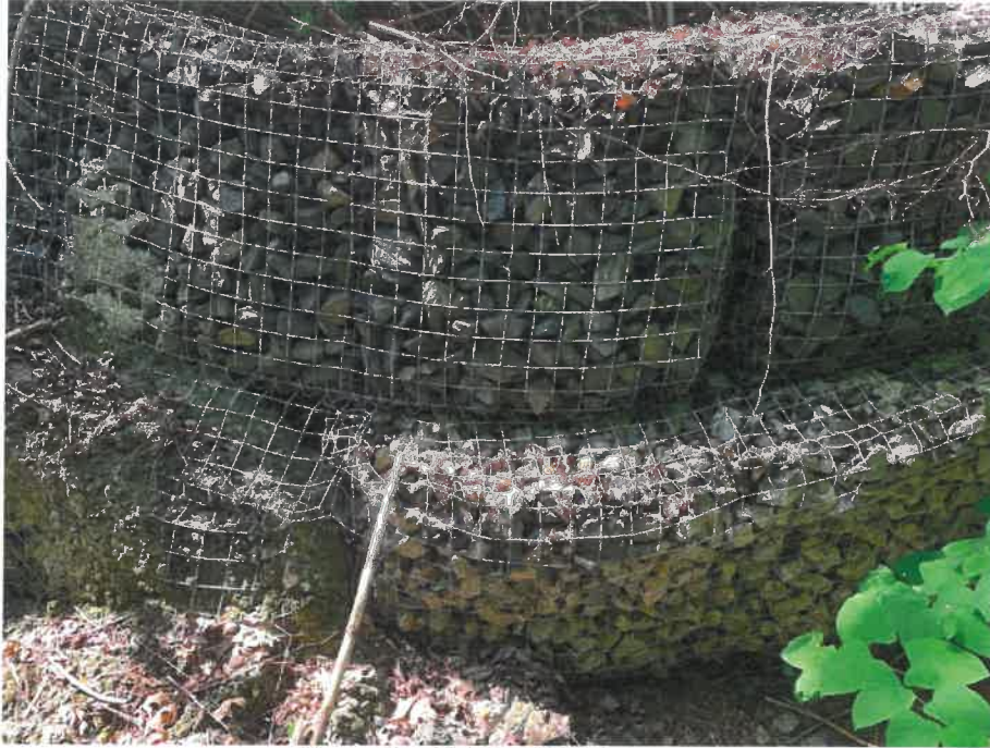
Figure 3 – Gabion Wall Closeup
