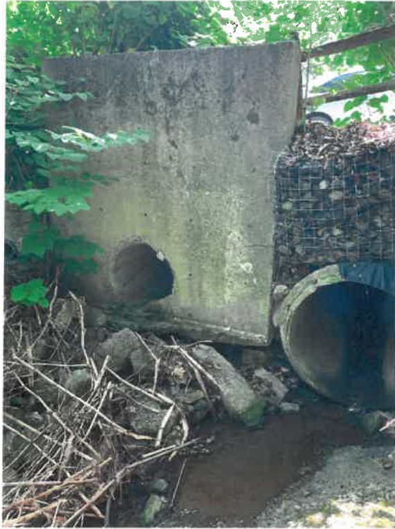
Figure 5 – Concrete Culvert Wall
